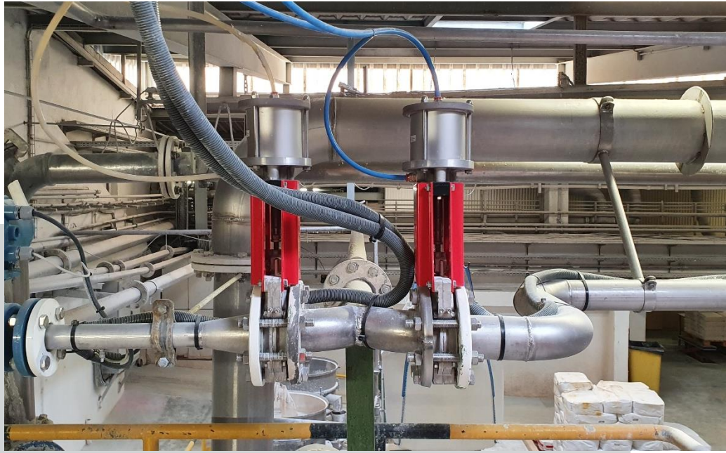
Wey knife gate valve VN in the dosing plant for calcium carbonate
