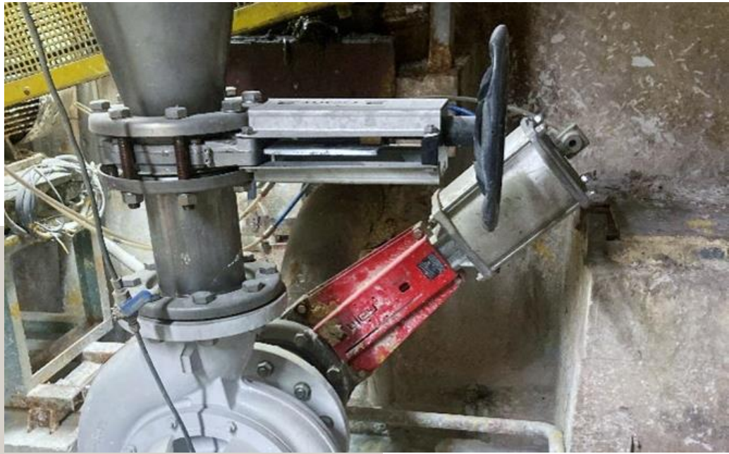
Manually and pneumatically operated Wey knife gate valves VN on the pulp pumps
