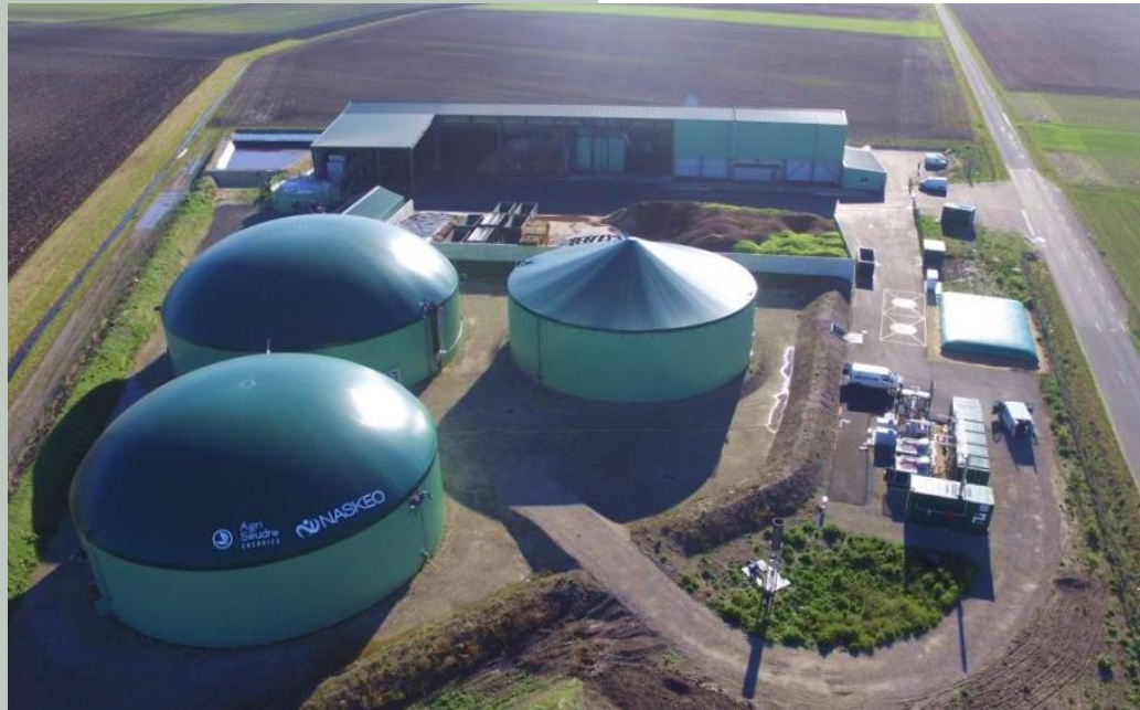
The newly built Agri Seudre Énergies biogas plant
